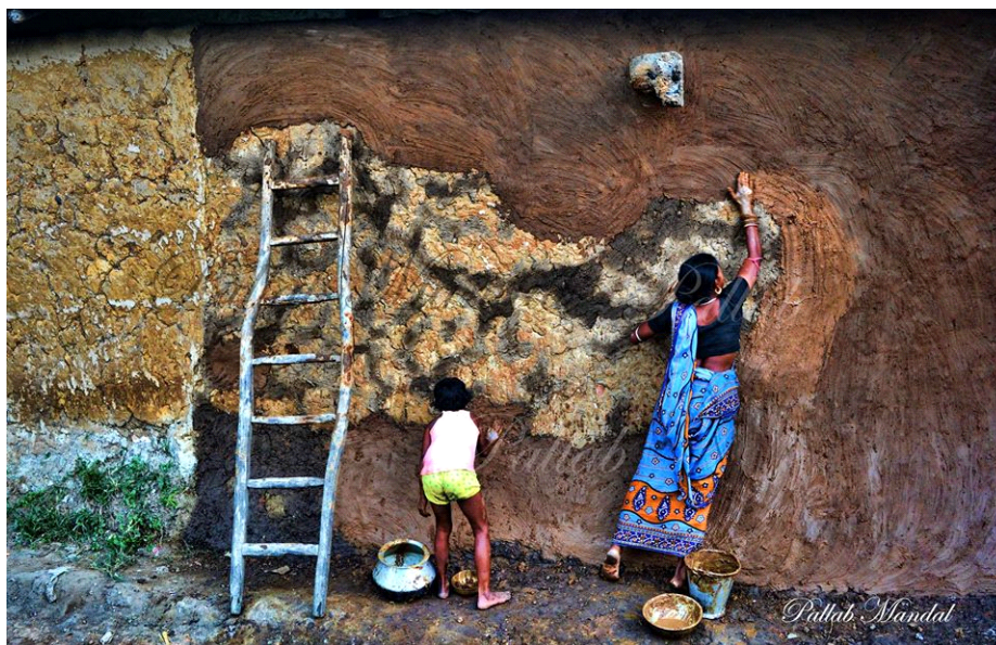
Figure 1: Renovation of the mud wall (Mandal, 2016, October 25).
